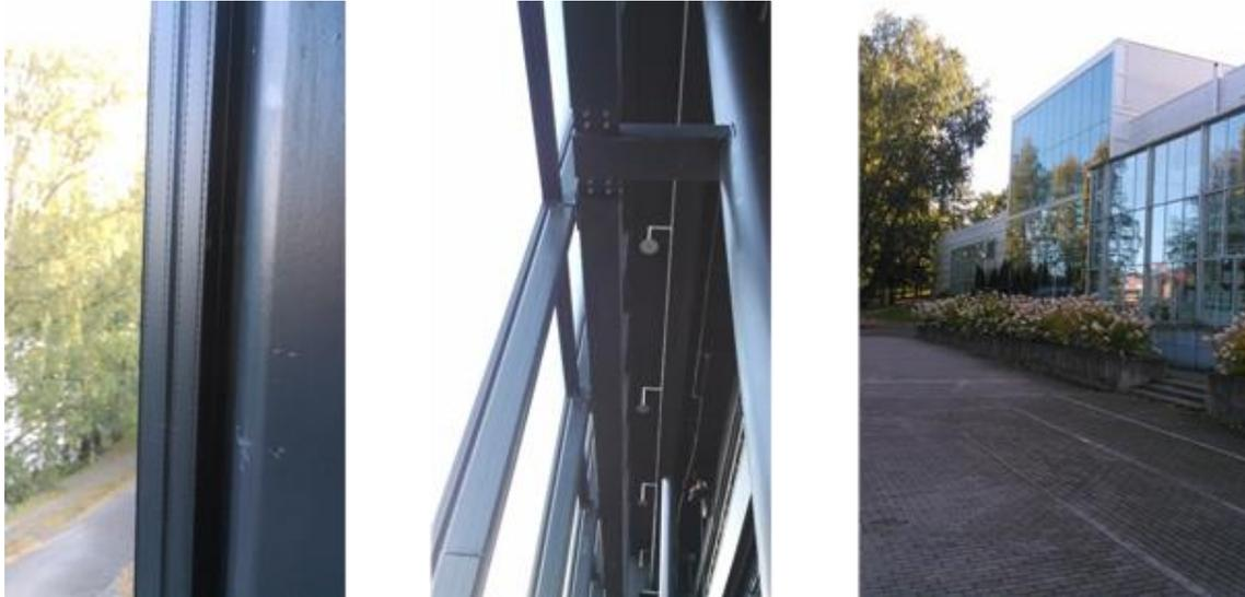
Figure 5 New glass facade of Tampere Concert Hall ( $U=0.8 \text{ W}/(\text{m}^2\text{K})$ )
